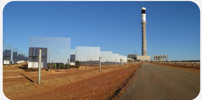
The 100MW Redstone concentrated solar thermal power (CSP) plant ^
