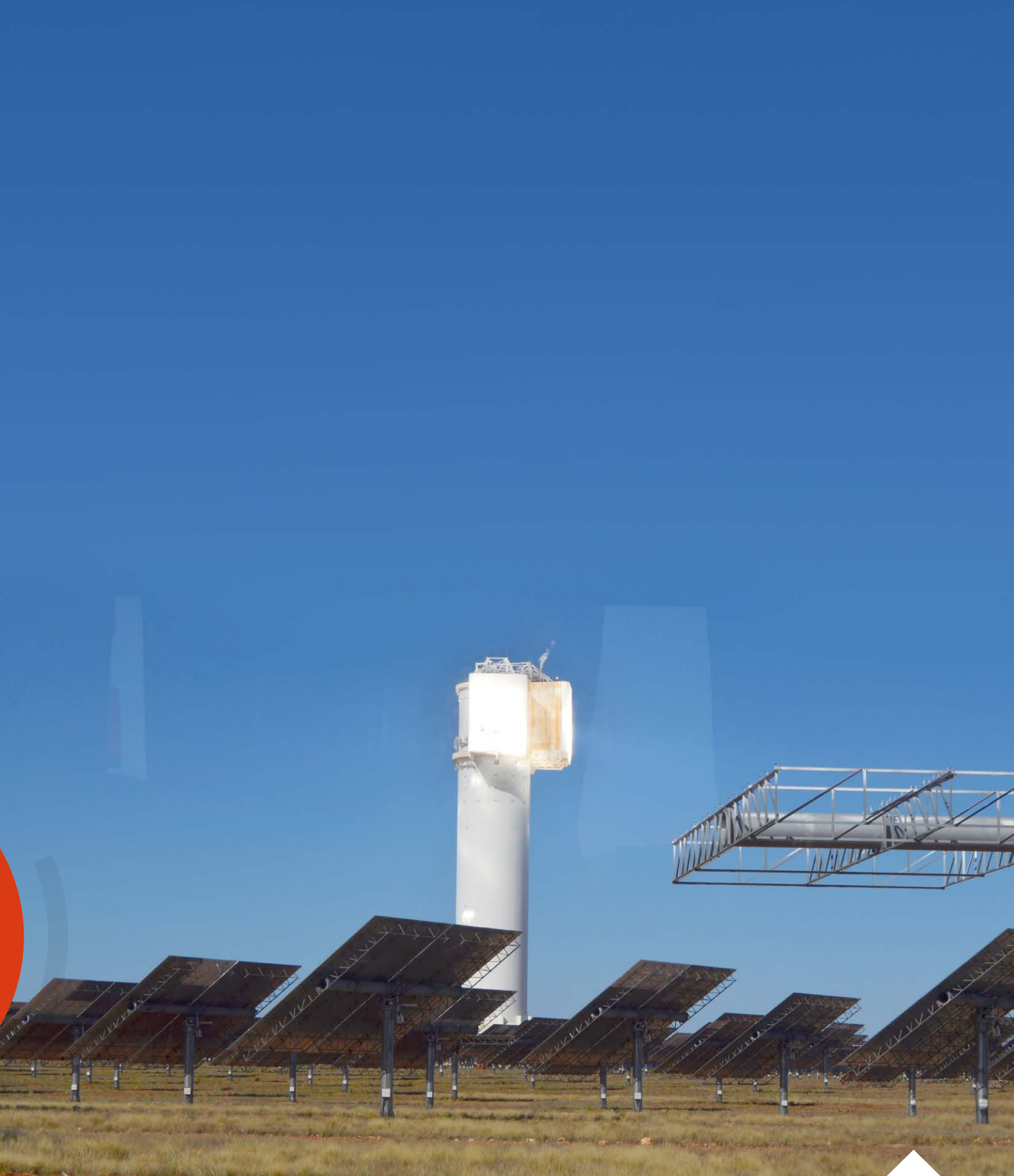
Khi Solar One -15MW CSP (Concentrated Solar Power) Plant
