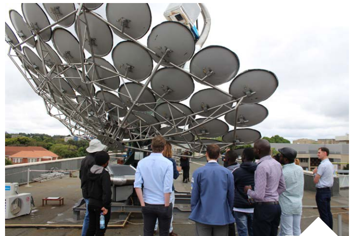
Viewing a solar dish installation
