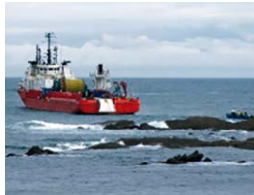
Cable installation at bimep
