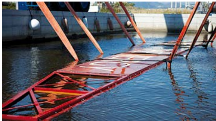
Installation R115 – 40 South Energy
