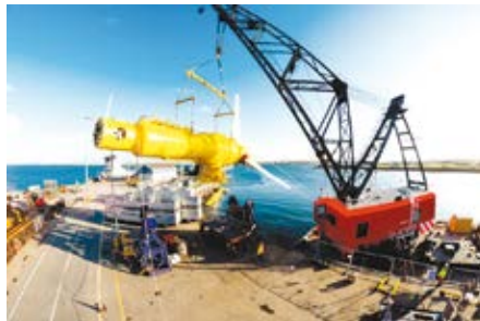
Alstom 1MW being lifted into water
