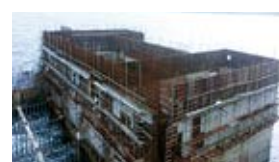
Construction of Yongsoo OWC Pilot Plant
