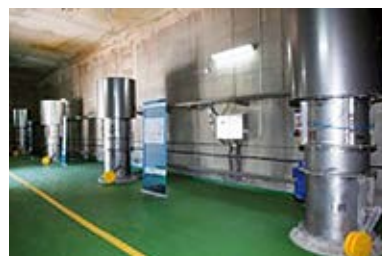
Turbines of the Mutriku OWC plant
