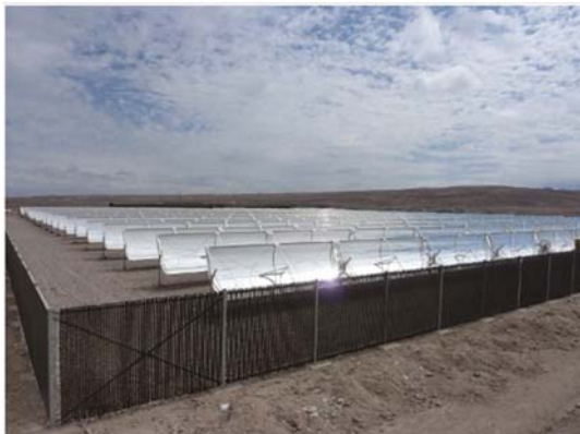
Abengoa. Installed plants
