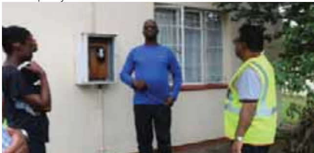
A customer with a newly installed Smart meter at Matatiele Local Municipality.
