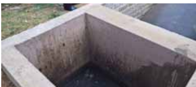
Completed biogas digester in Sharpeville with biofertilizer.
