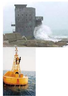
According to the IEA GIEC has been researching shoreline, concrete OWC systems since 1985. Their first device was rated at 1kW and was followed by a 20 kW system. In 2001 a 100 kW demonstration plant was deployed in the Guangdong Province and was grid connected for 2 years. GIEC also developed 5 kW floating, offshore OWC called a backward bent duck buoy.
