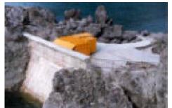
In 1983 the Sanze shoreline gully was constructed. It is a 40 kW shoreline OWC consisting of steel and concrete. It functioned for several years before it was decommissioned and inspected for corrosion and fatigue.
