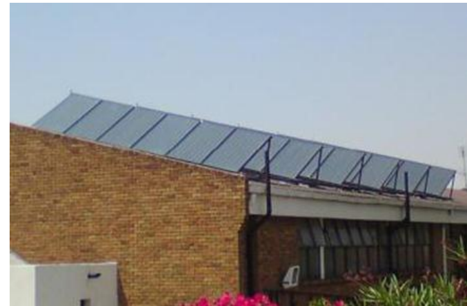
System 4 at ABI Miller , North Riding
