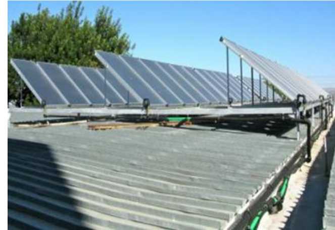
System 6 Katutura State Hospital , Windhoek
