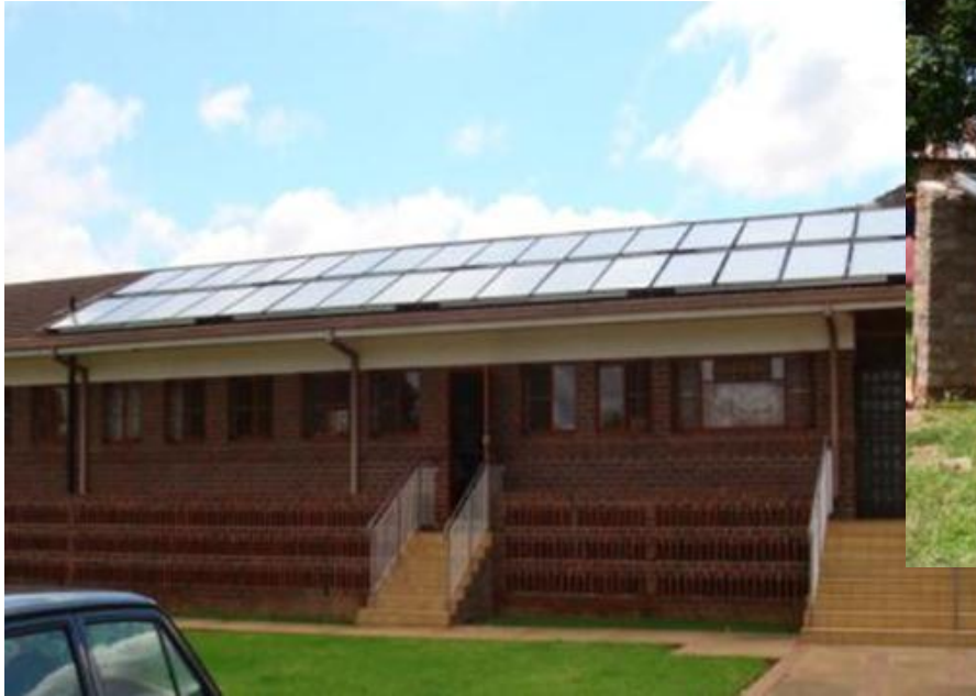
Pumped system - home of retired sisters, Zimbabwe
