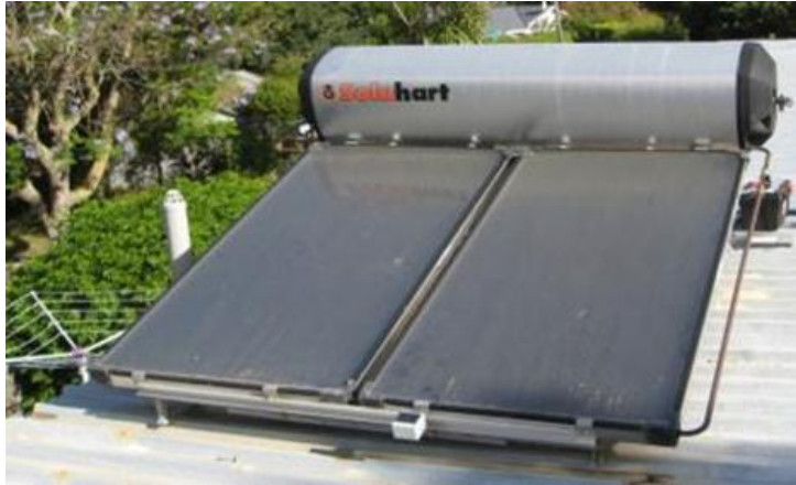
System 1 at a commercial laundry , Cape Town
