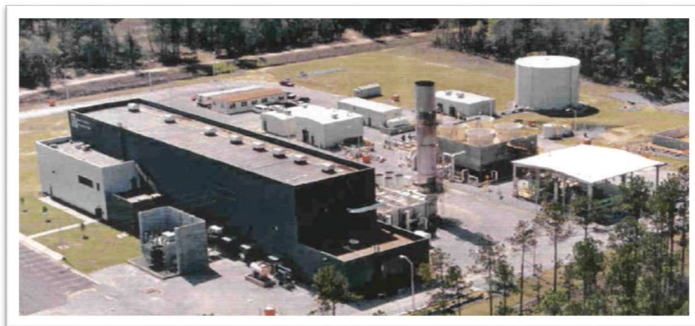
Aboveground facilities for 110-MW McIntosh Alabama CAES plant
