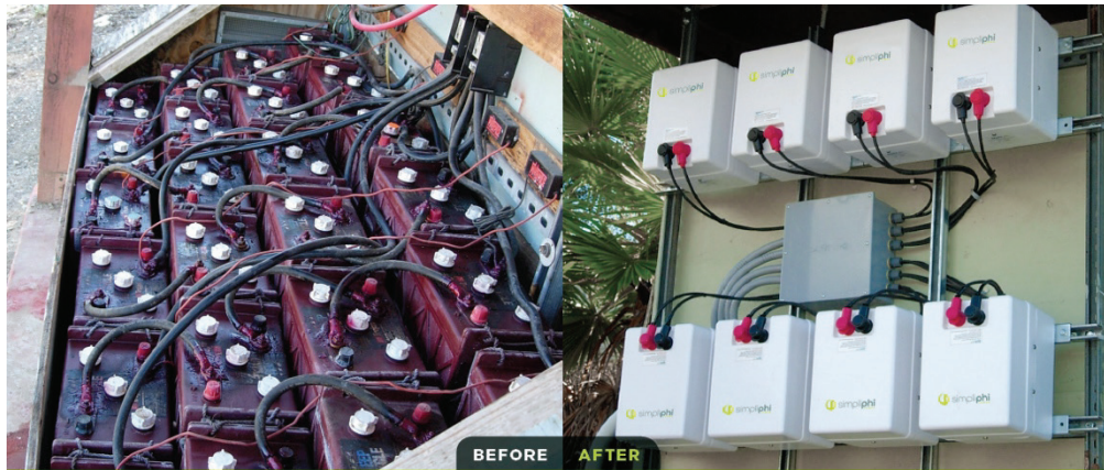
Example: SimpliPhi of drop-in replacement capability.
