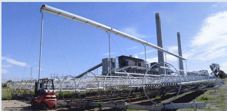
Figure 4-3: CFLR installation at the Liddell power plant.
