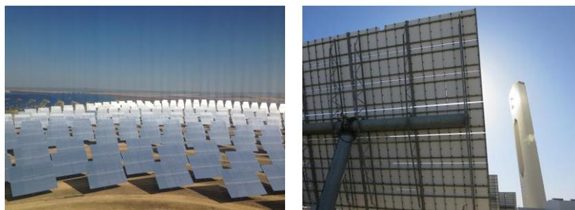
Figure 6: Heliostats in the field (left) and the cavity receiver in operation (right) at PS20, Spain
