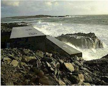
The limpet is designed by Wavegen; a unit has been operational in Islay (an island off Scotland's west coast) where it supplied electricity to the national grid. The limpet operates on the owc (waves causes an air pocket, which is trapped behind a wall, to oscillate) principle and it uses a Wells turbo generator that drives an induction generator in order to convert the extracted energy into electricity.
