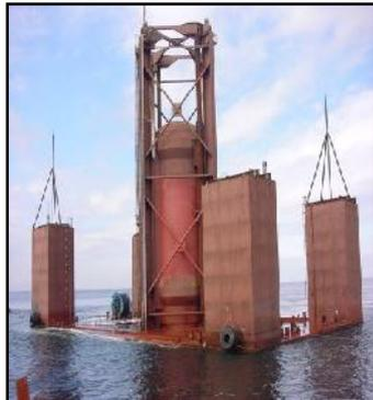
It consists of two cylinders the lower one is fixed to the seabed and the upper one is allowed to move swell. An air pocket is trapped inside the upper cylinder; this pocket is compressed when the peak of the wave passes. This forces the float down, thereby compressing the air, when the trough passes the compressed air forces the float back up. This causes the float to oscillate.
