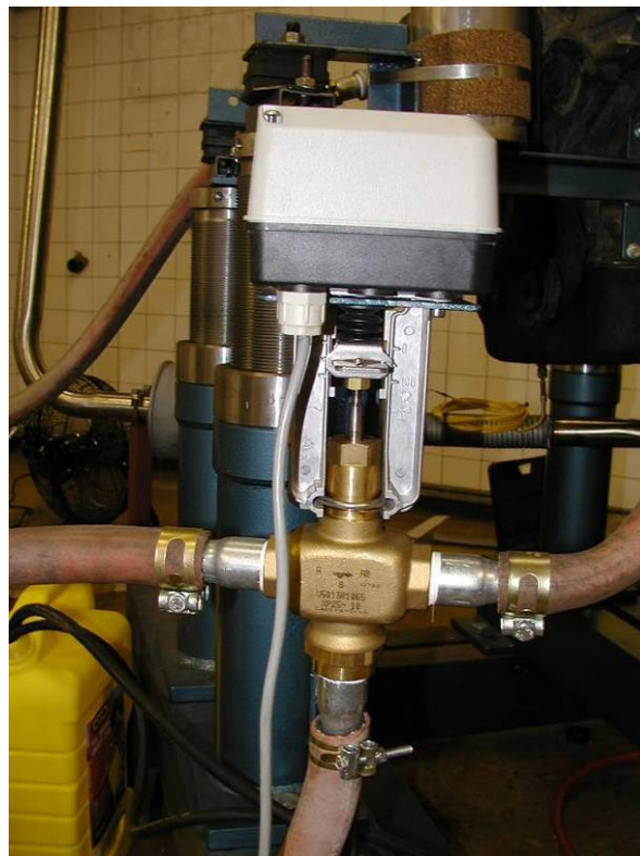
Figure 3-12: 3-way valve actuator
