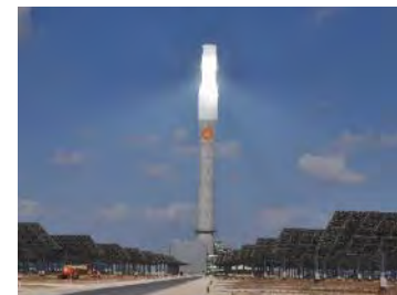
Gemasolar, molten salt, 19 MW e , Spain, 2011
