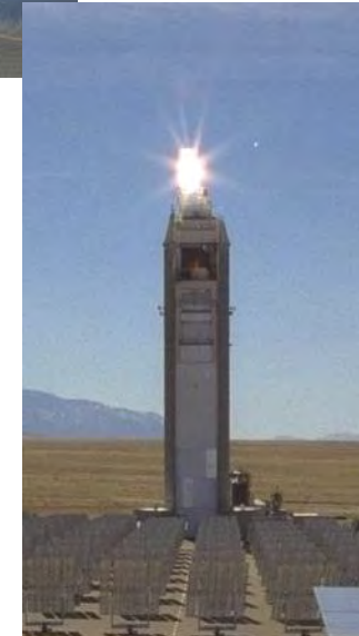
Thermal emission from receiver at ~600 C
