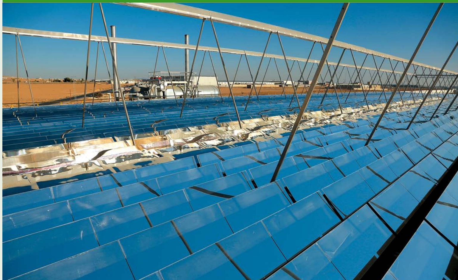
Linear Fresnel collectors used for direct steam generation for the solar cooling system at the Japan Tobacco International factory in Jordan.
