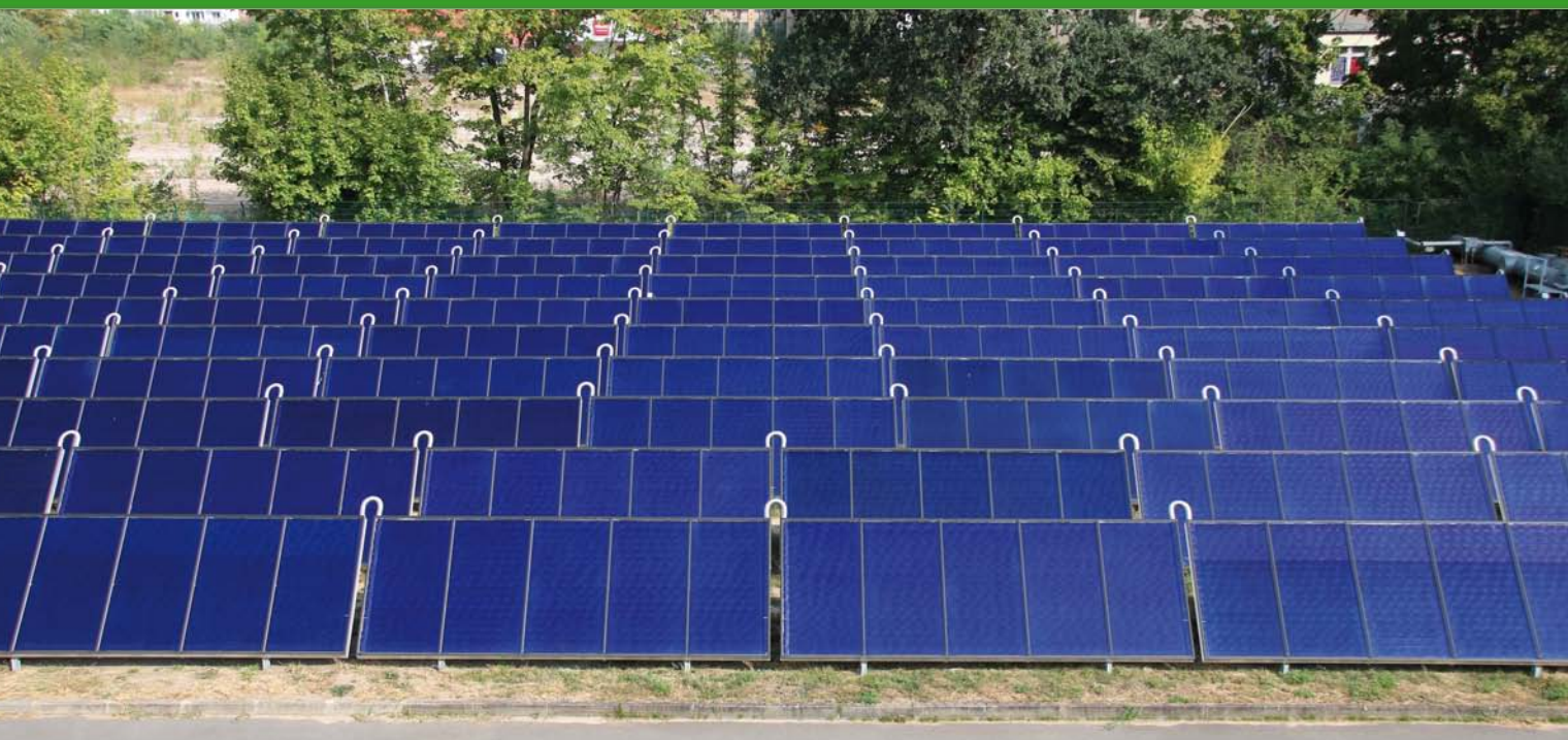
A 0.7 MW th solar thermal system supplies heat to the Berlin district heating network.
