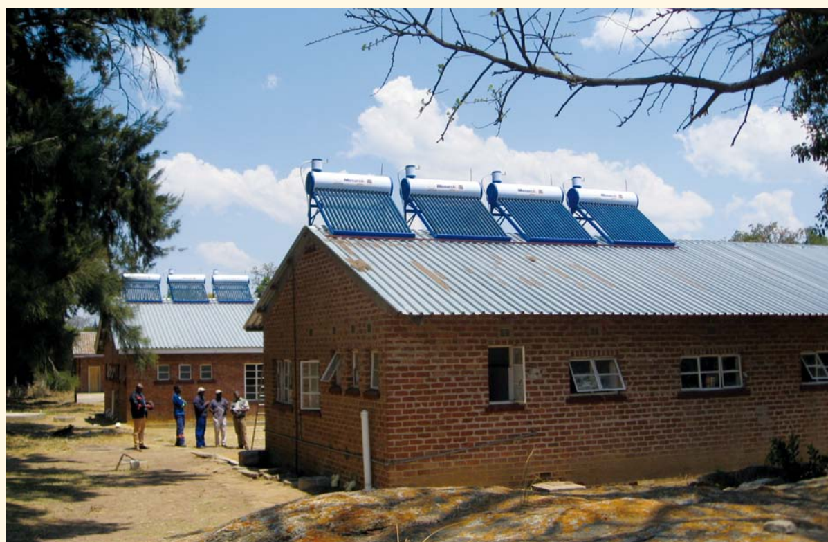
Demonstration system at Matopo Highschool in Zimbabwe with a collector area of 13 m 2 .
