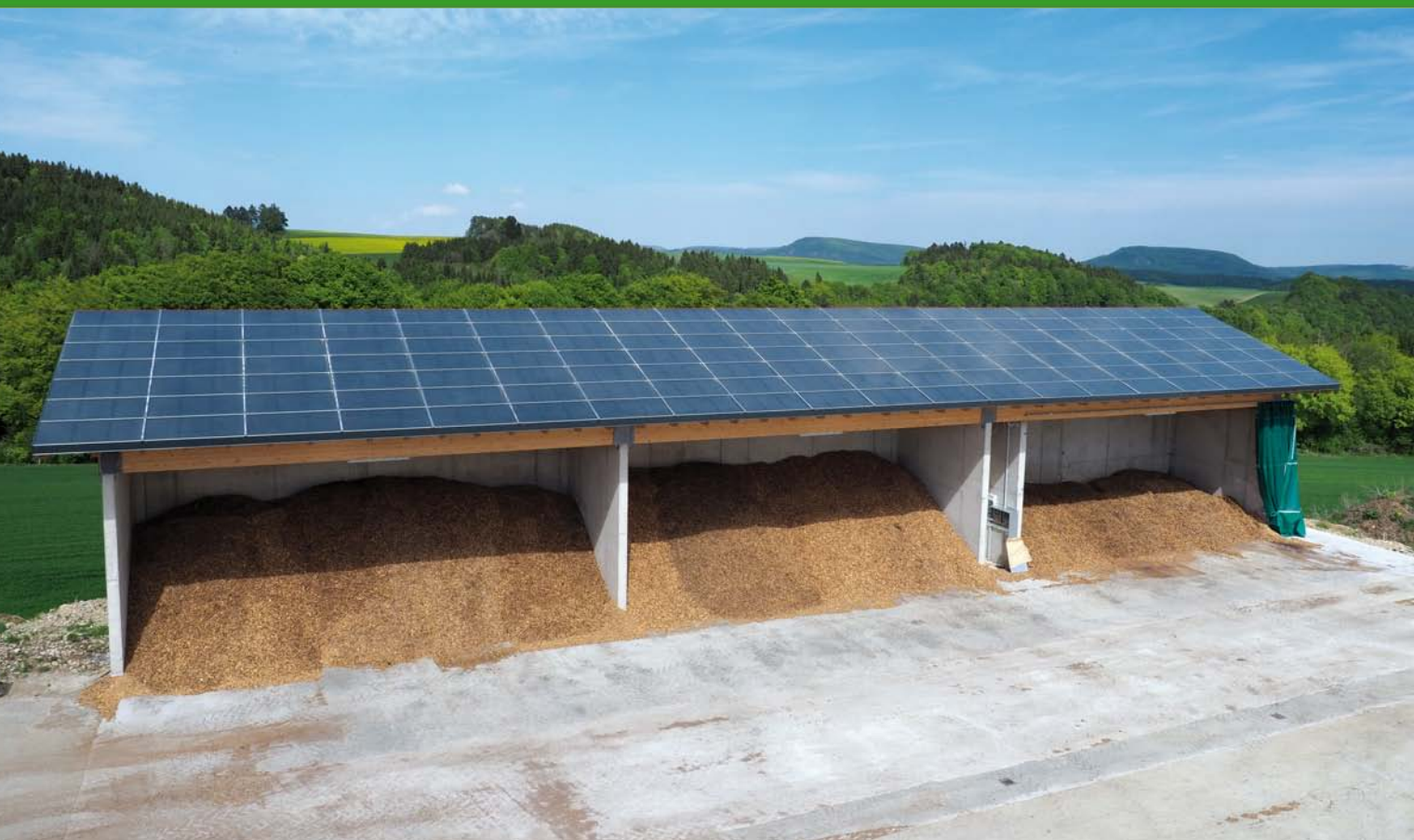
A 224 m 2 solar air collector field is used for commercial woodchips drying in Edlbach, Austria.
