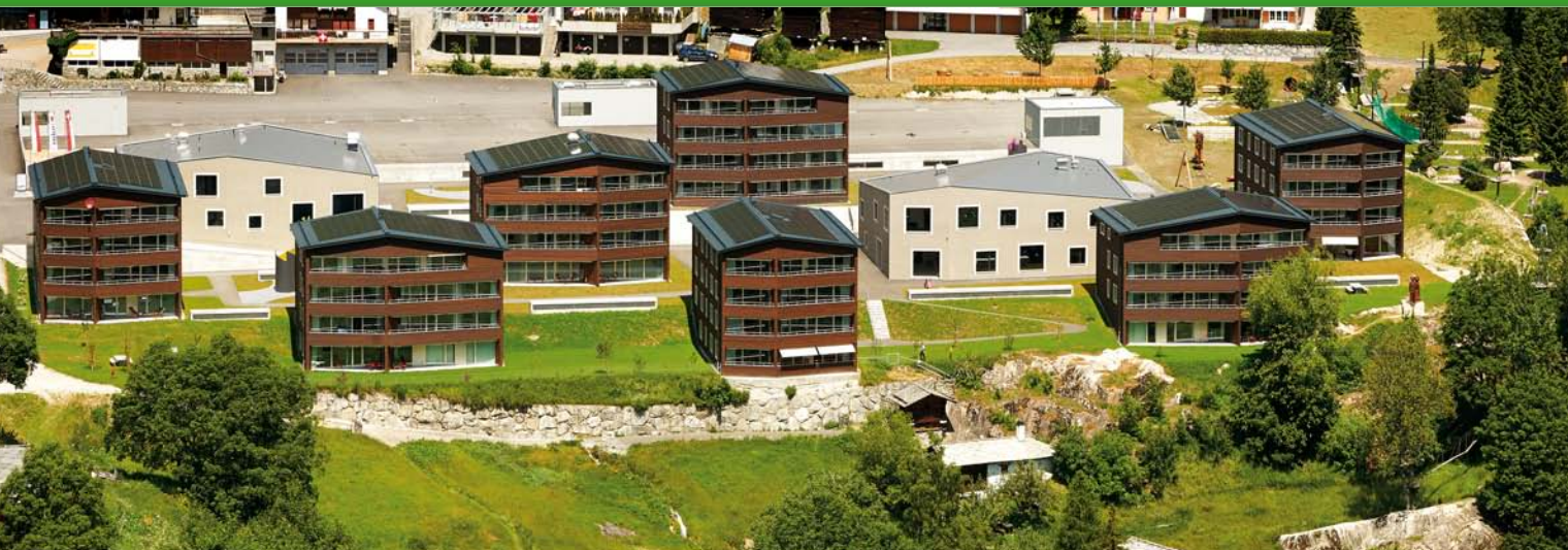
672 m 2 uncovered PVT collectors in Switzerland.
