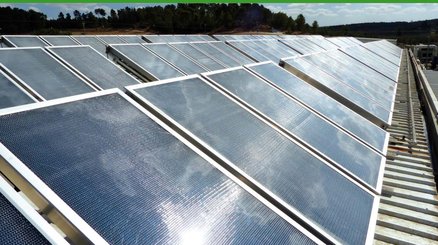
Flat plate collectors with transparent insulation used for a cleaning process in an Israeli dairy.
