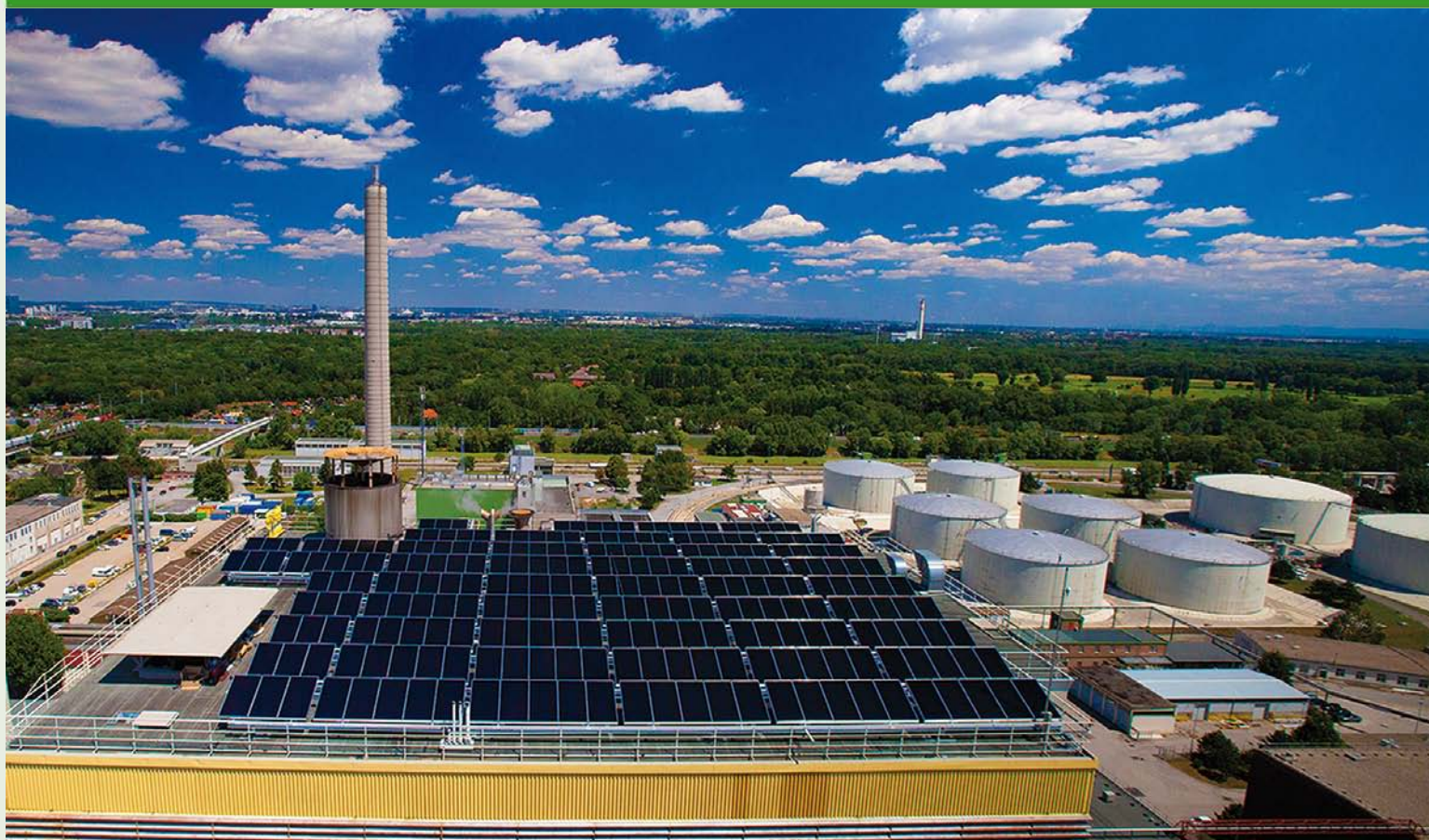
In Vienna 656 m 2 flat plate collectors were installed on the roof of a boiler house at a height of 70 meters. Photo: Greenonetec Solarindustrie GmbH
