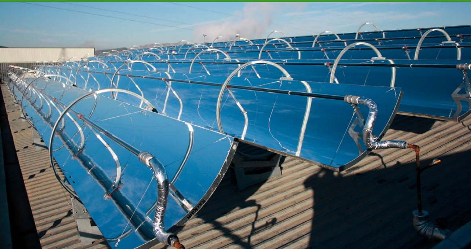
The food-processing plant of the company Papes Safor in Spain uses parabolic trough collectors.
