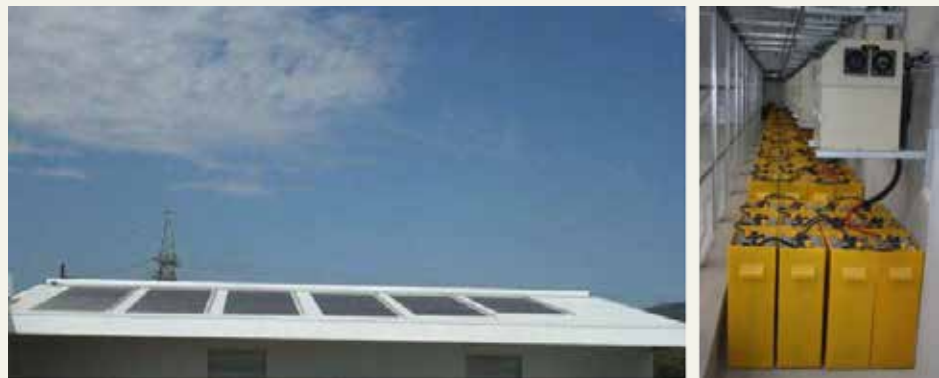
Figure 7: The 30kW p PV installation at IMPERIAL Cargo with battery storage
