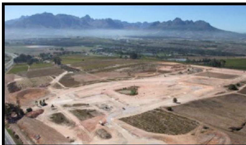
Figure 4.8 The construction of Longlands Estate, currently underway
