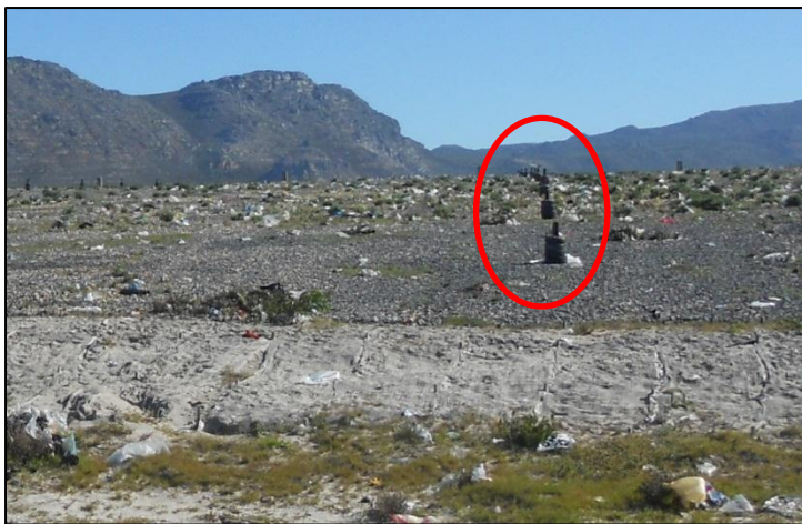
Figure 6: Gas pipes at Coastal Park Landfill
