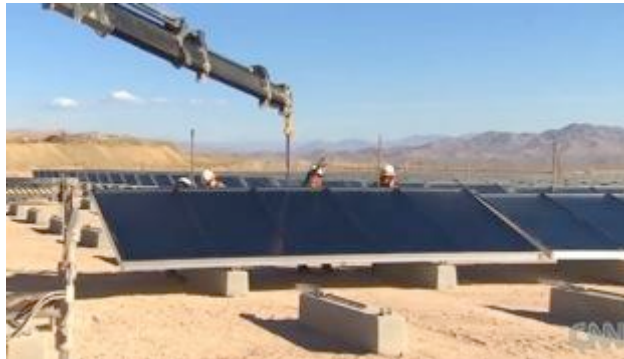
Figure 7: The world's largest solar thermal installation for industrial application at a copper mine in Chile 43
